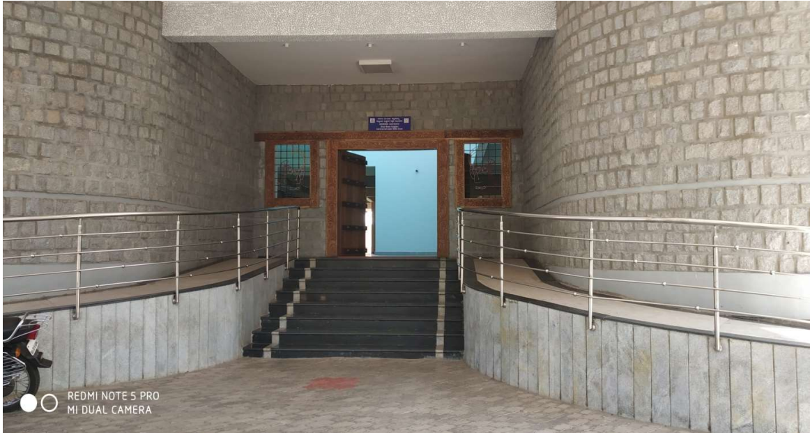
Nudi (class room complex)-Ramp
