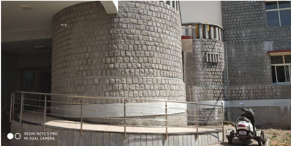
Nudi (class room complex)-Ramp
